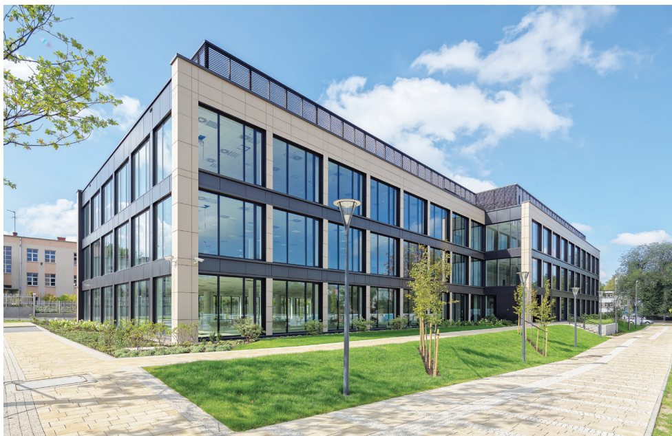
Fot: Radom Office Park
